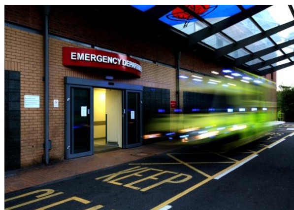
University Hospital North Durham A&E department
